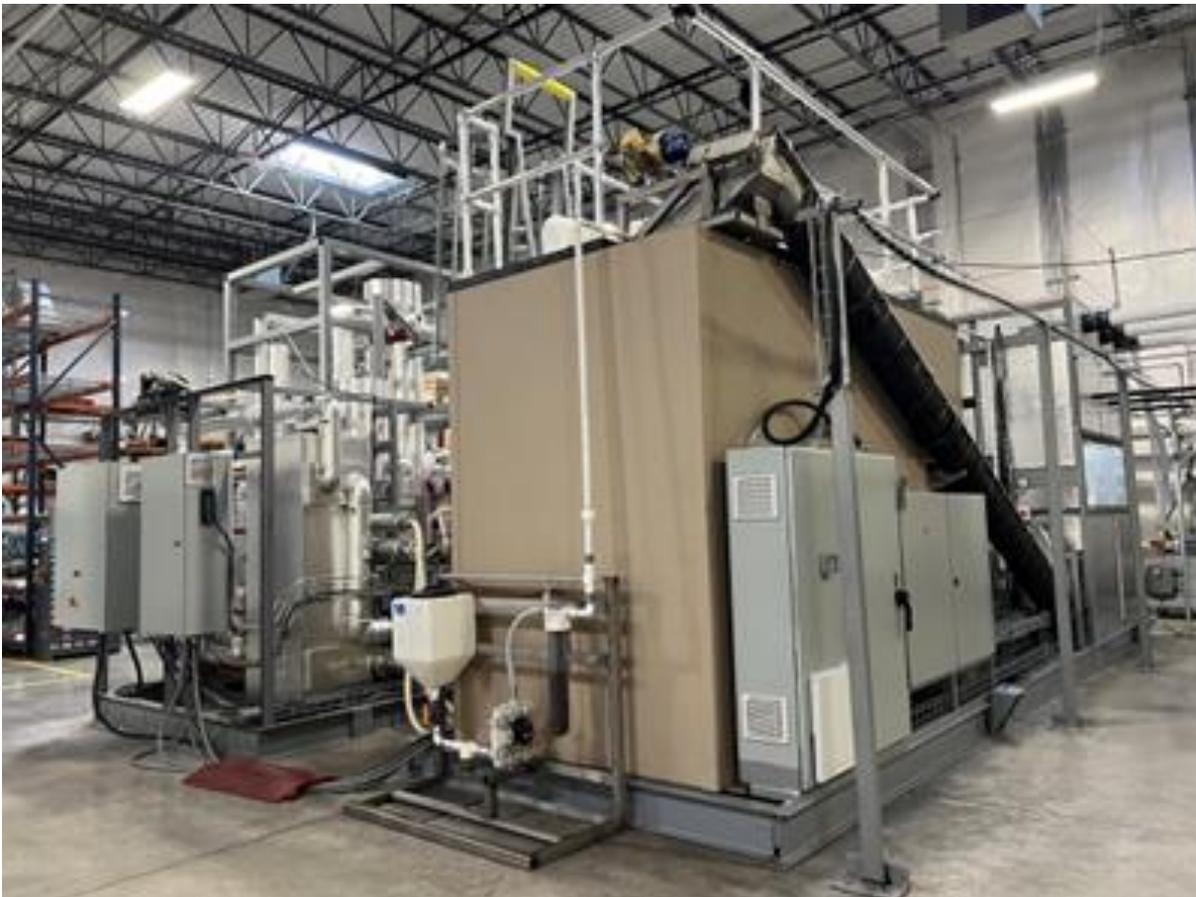
**Figure 2: the current 100kW<sub>th</sub> commercial unit at Rebound's facility in commerce city CO. (left) ice storage tank (right) separation system, our test cell can simulate a 100,000+ sqft. cold chain facility.**
