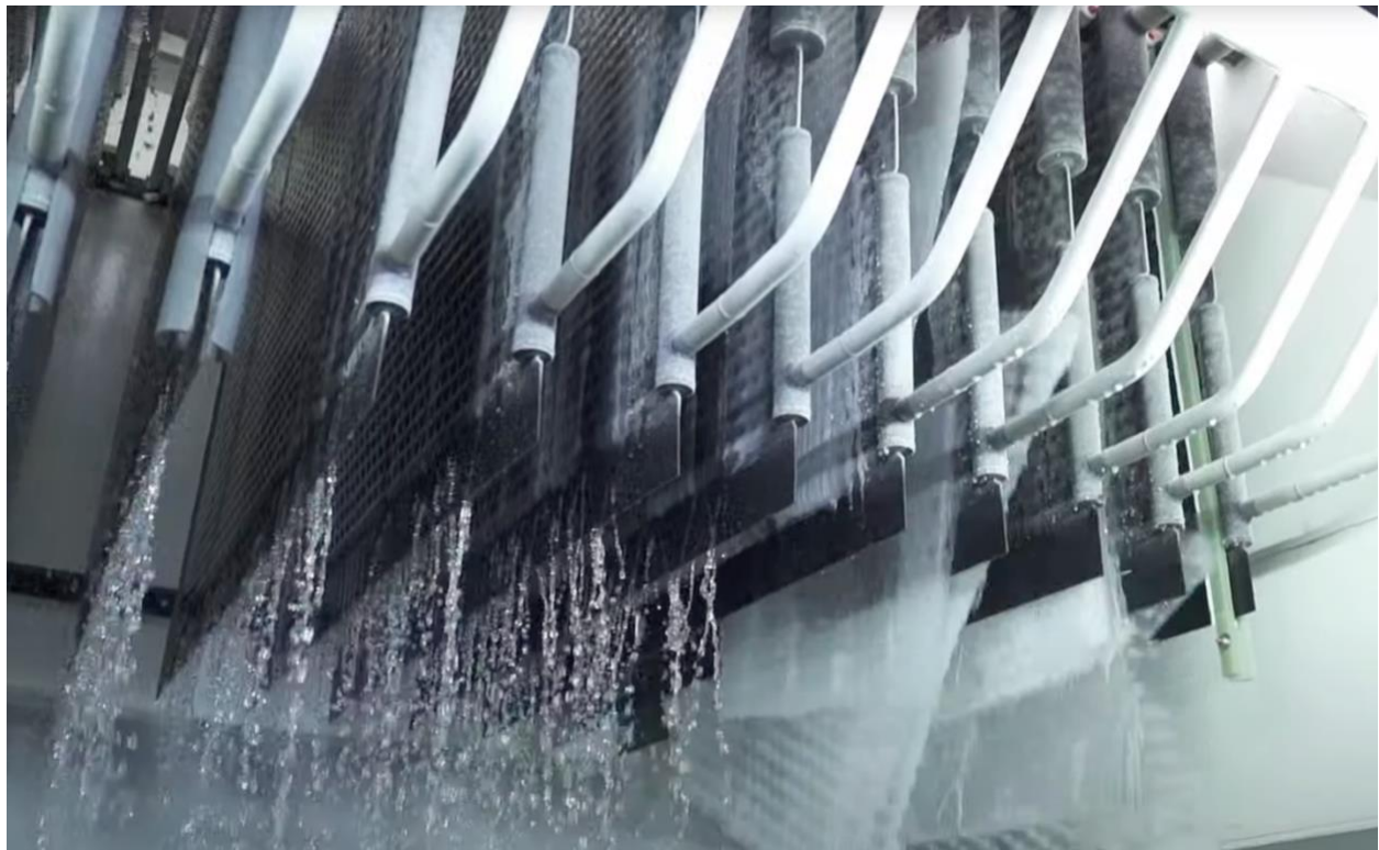
Figure 2: The IcePoint system in action. System controls are very similar to a falling film chiller, with harvest triggered by the curtailment of water flow.
